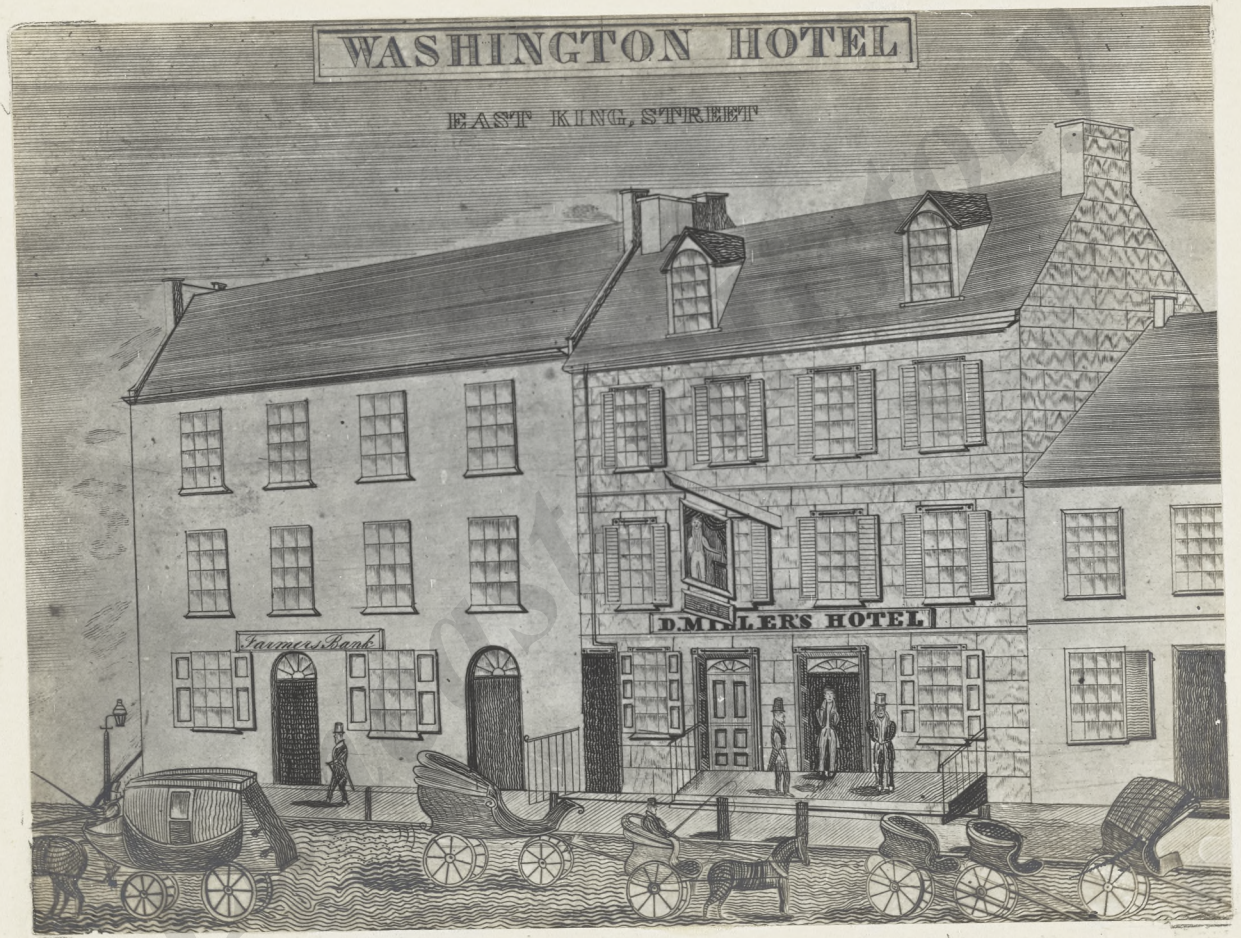
David Miller's Washington House - S. side King W. of Duke St.
