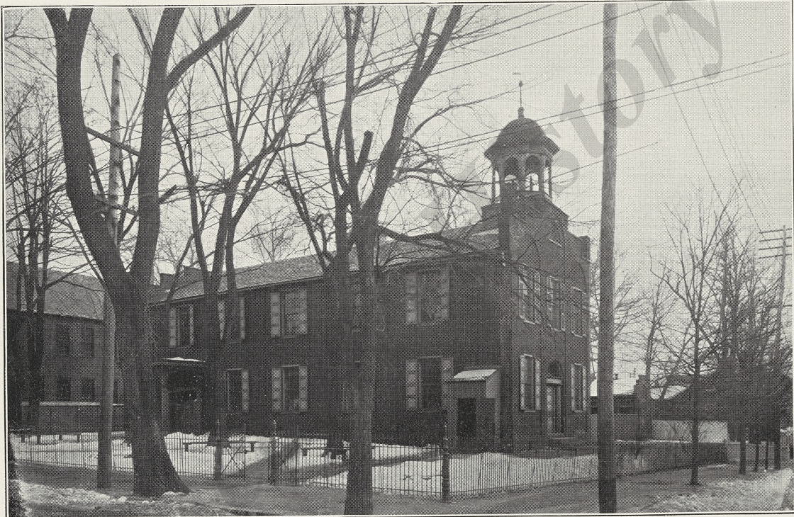
LANCASTERIAN SCHOOL BUILDING.
