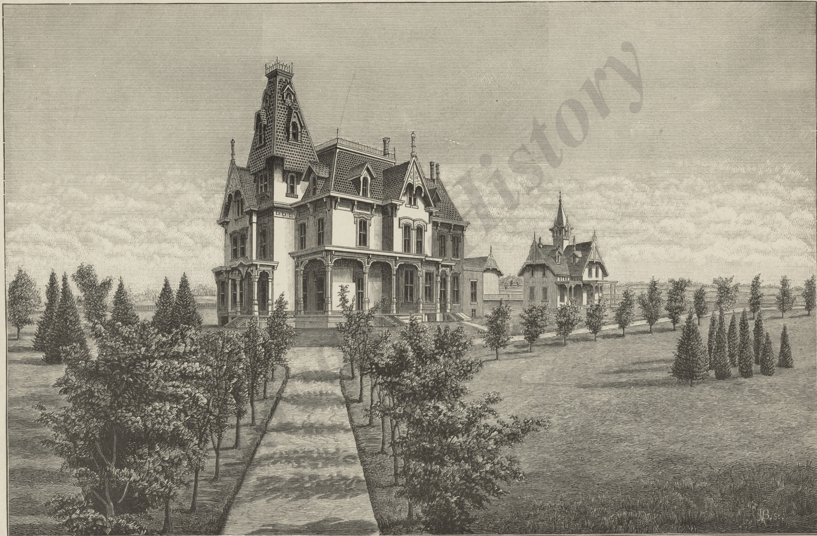
RESIDENCE OF COL. L. L. BUSH, BIRD-IN-HAND, LANCASTER CO., PA.
