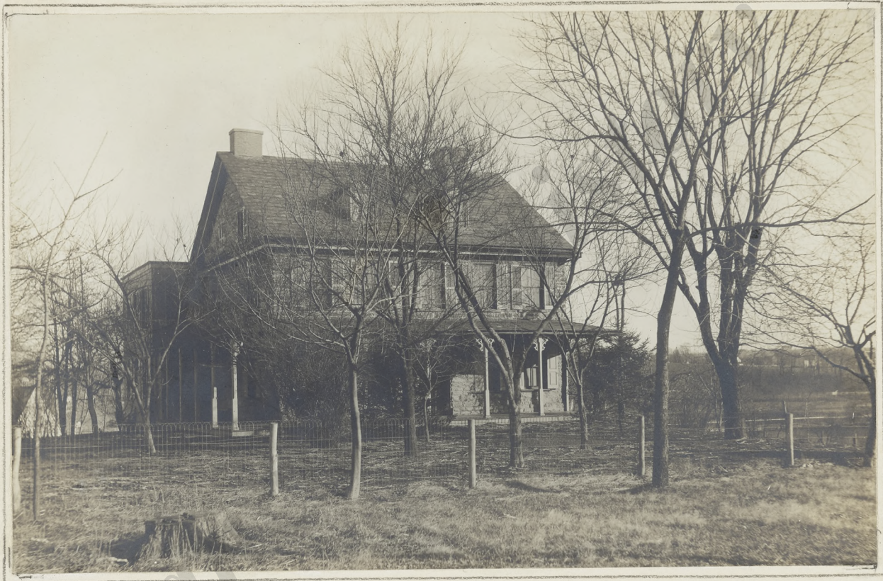
Dwelling House at Ranck's Mill.
