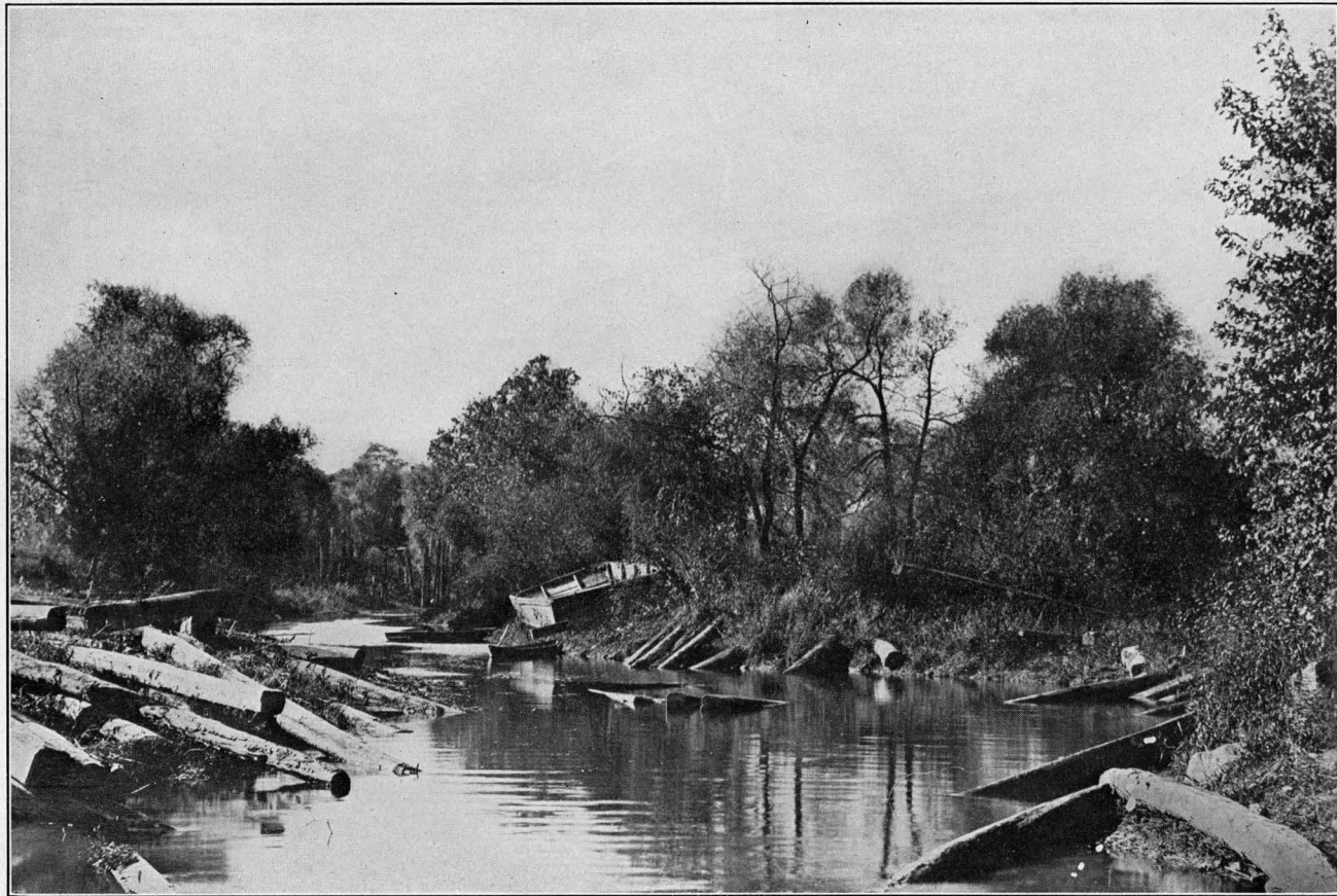
Bed of Susquehanna and Tidewater Canal at Wrightsville, Pa., now used as a Saw Mill Dam.
