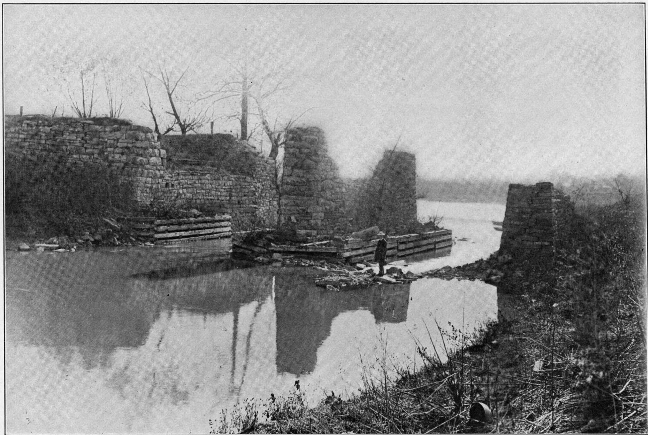
Ruins of Kishacoquillas Creek Aqueduct, at Lewistown, Pa.
