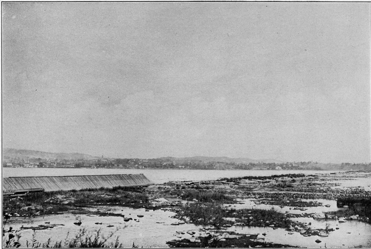
Ruins of Columbia Dam, Columbia, Pa.
