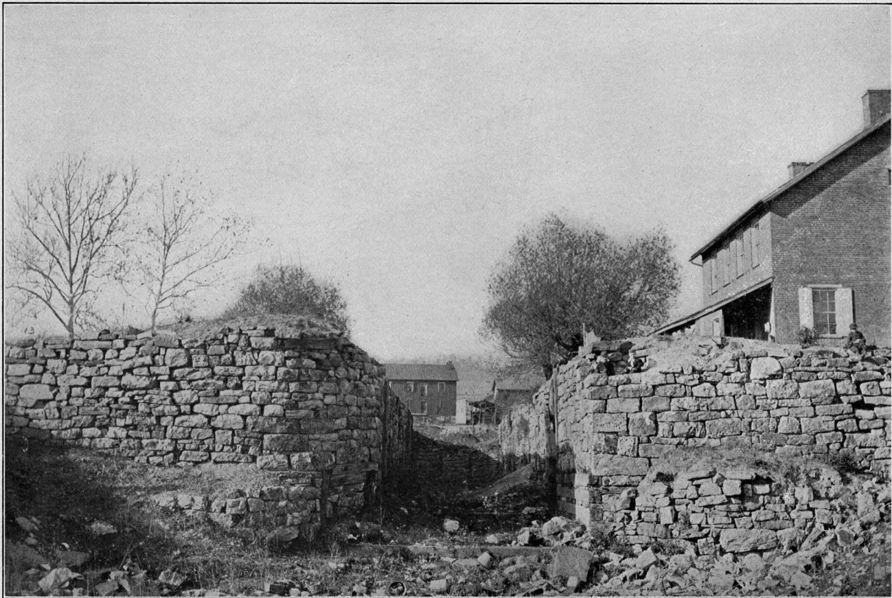
Ruins of Lock on Juniata Division, Pennsylvania Canal, at Lewistown, Pa.
