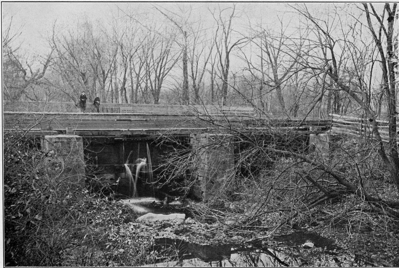
Canal Aqueduct crossing Fishing Creek, at Fort Hunter, Pa.
