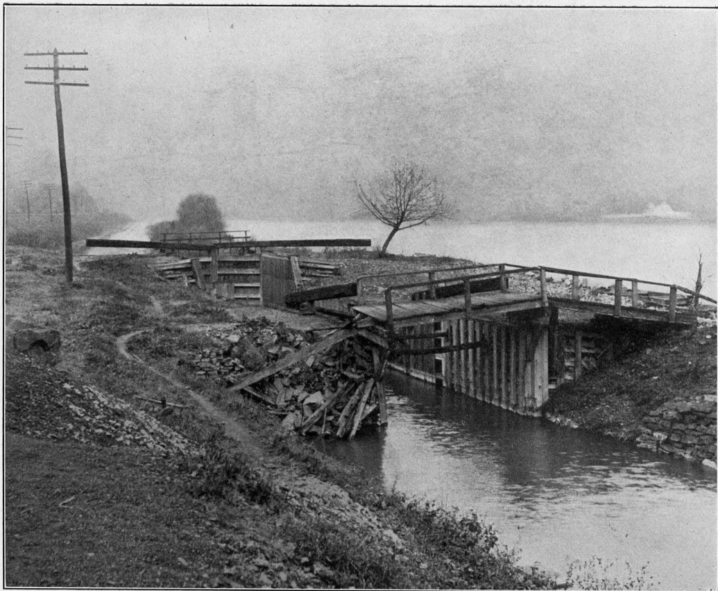
Abandoned inlet lock, Old Ferry Station, Pa.
