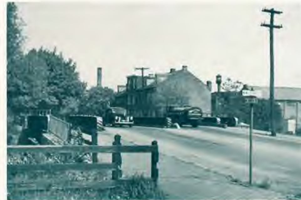
Figure 71. Hazardous obstruction on an arterial street.
