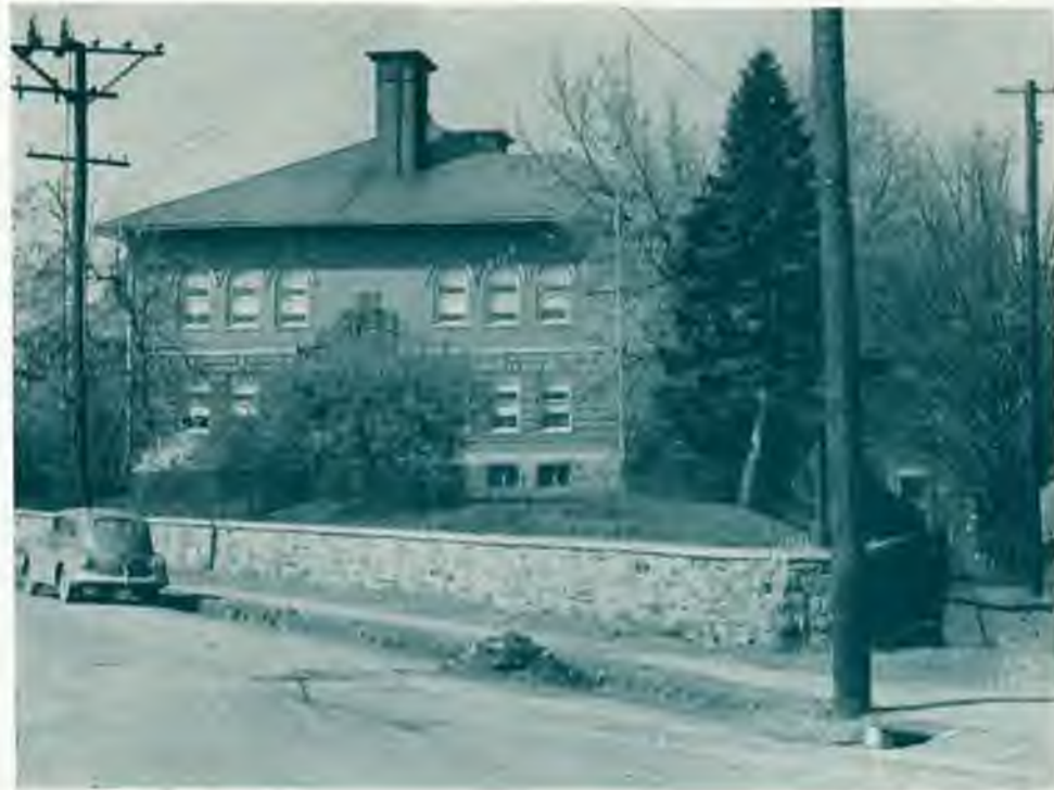
Figure 49. Buehrle Elementary School—50-year-old structure on inadequate site.
