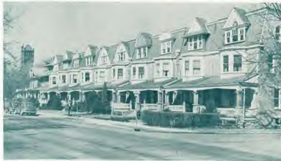
Figure 27. Substantial row houses in a conservation neighborhood.
