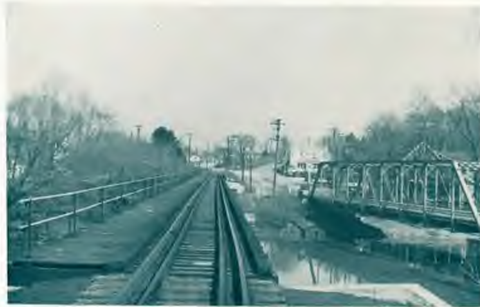
Figure 69. Route 222, South-City approaches need improvement.
