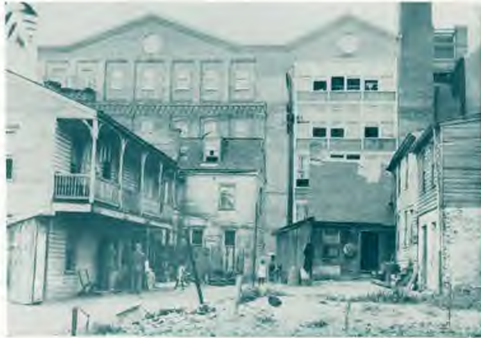
Figure 23. Dunie's Court—A community hazard.
