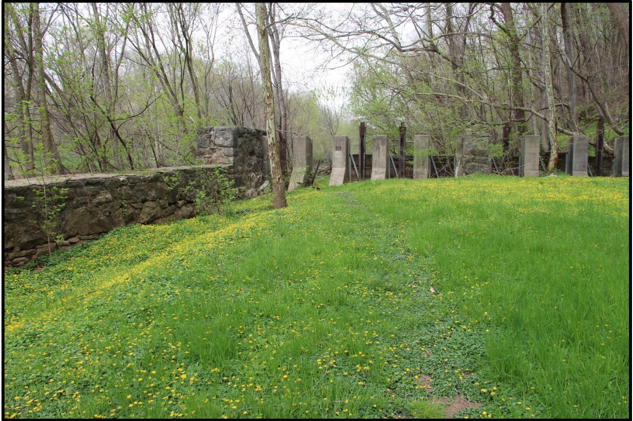
Photo 6: View of ruins of Lock No. 5 at Rockville, Pennsylvania, facing north. Remnant of historic-age lock wall is visible at left. Sluice gates at center and right date to a twentieth-century conversion of the lock and dam for water power generation.
