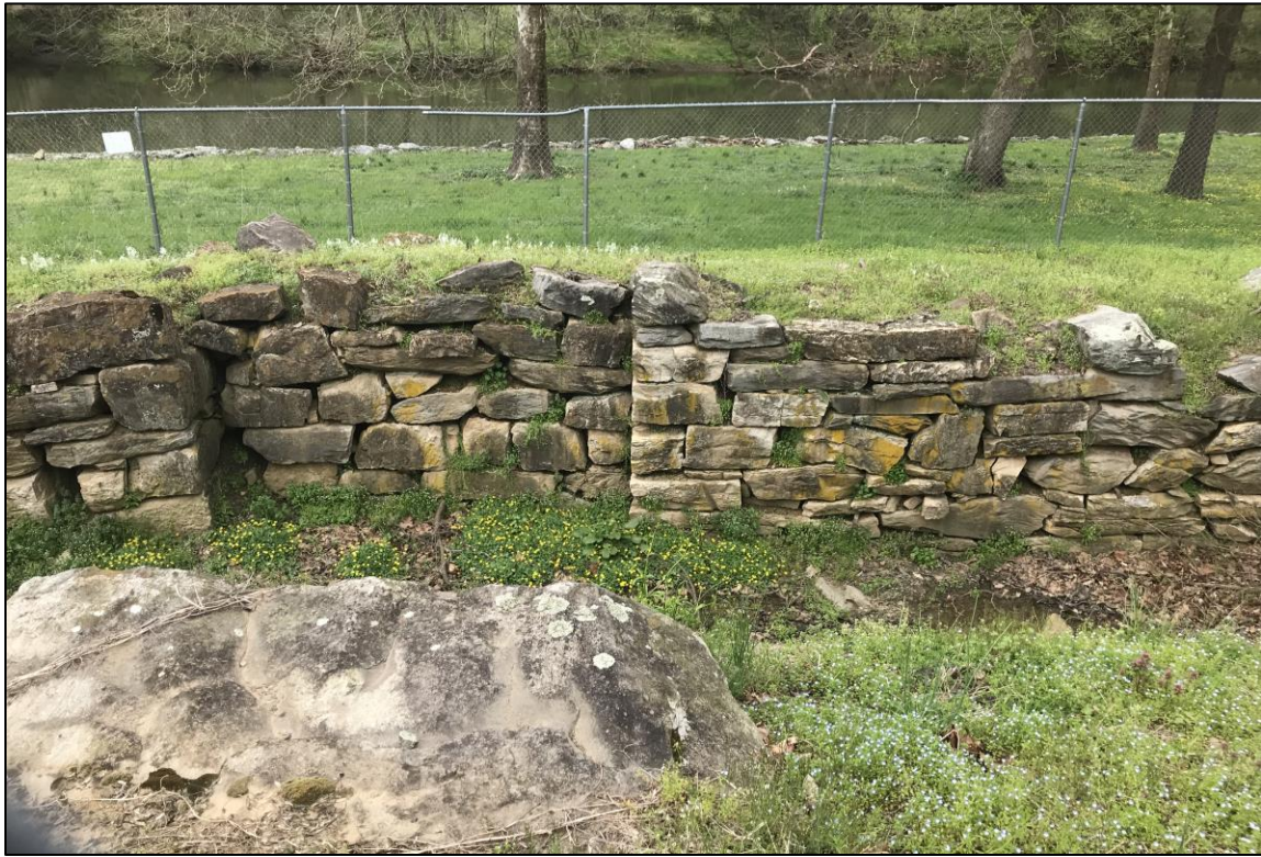
Photograph 5: Detail, west wall of Lock No. 6 (Lock No. 8), facing northwest.
