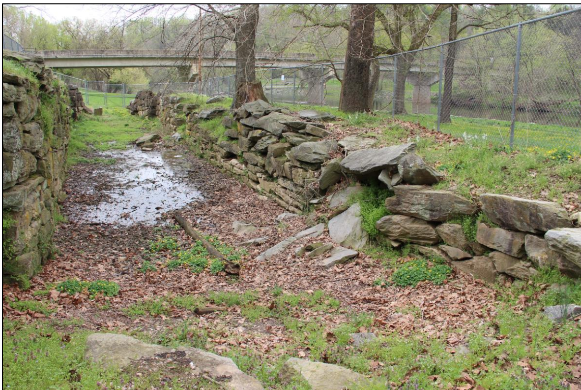
Photograph 3: Detail, Lock No. 6 (Lock No. 8), facing southwest.
