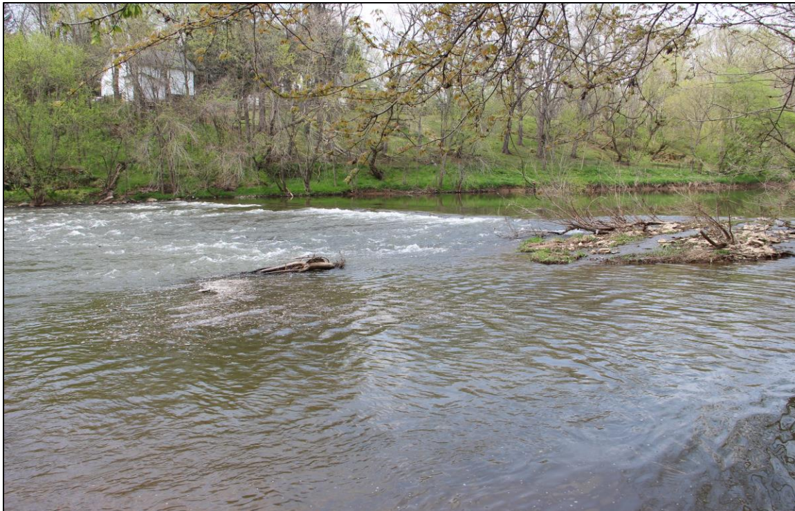
Photograph 10: Detail, Lock No. 5, showing ripples in Conestoga River, location of twentieth century hydroelectric dam (demolished), facing northwest.
