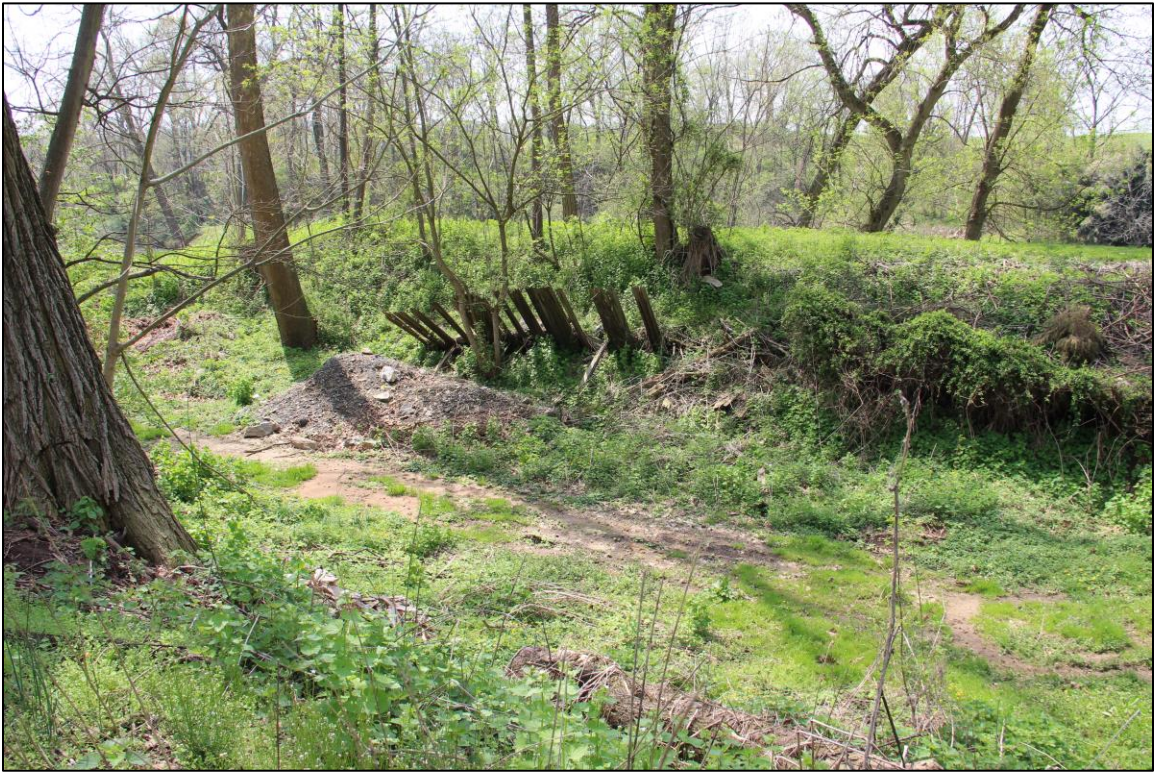
Photograph 13: Detail, Lock No. 4 sluiceway, facing northwest. Age and association of wooden features (middle) are unknown.
