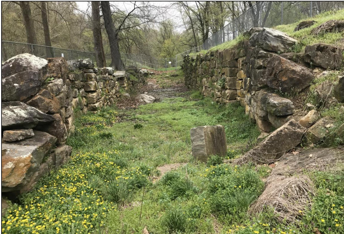
Photograph 6: Detail, Lock No. 6 (Lock No. 8), showing lock chamber, facing north.
