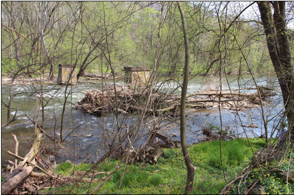
Photograph 16: Overview, Lock No. 1, showing twentieth century dam (demolished) from west embankment of Conestoga River, facing southeast.
