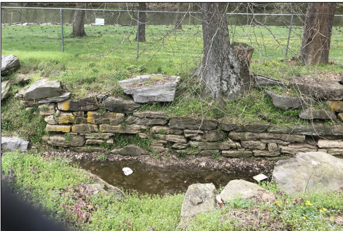
Photograph 4: Detail, west wall of Lock No. 6 (Lock No. 8), facing northwest.
