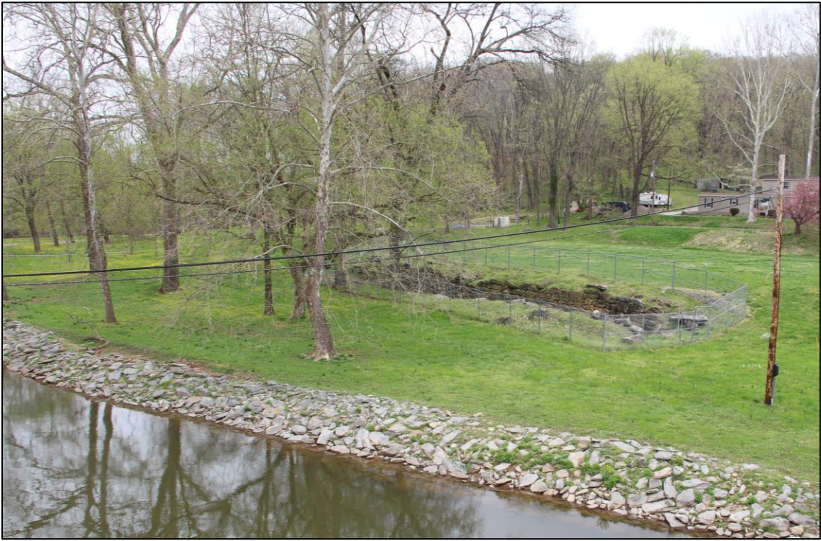
Photograph 1: Overview, Conestoga Navigation Lock No. 6 (Lock No. 8) showing ruins of lock and relationship to Conestoga River. Note river embankment reinforced with rip rap. View from River Road (SR 3017) Bridge, facing northeast.
