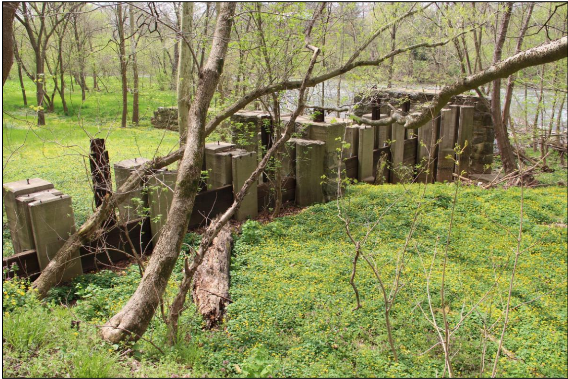
Photograph 9: Detail, Lock No. 5, twentieth century sluice gates (foreground) and altered west wall of lock (background), facing southwest.
