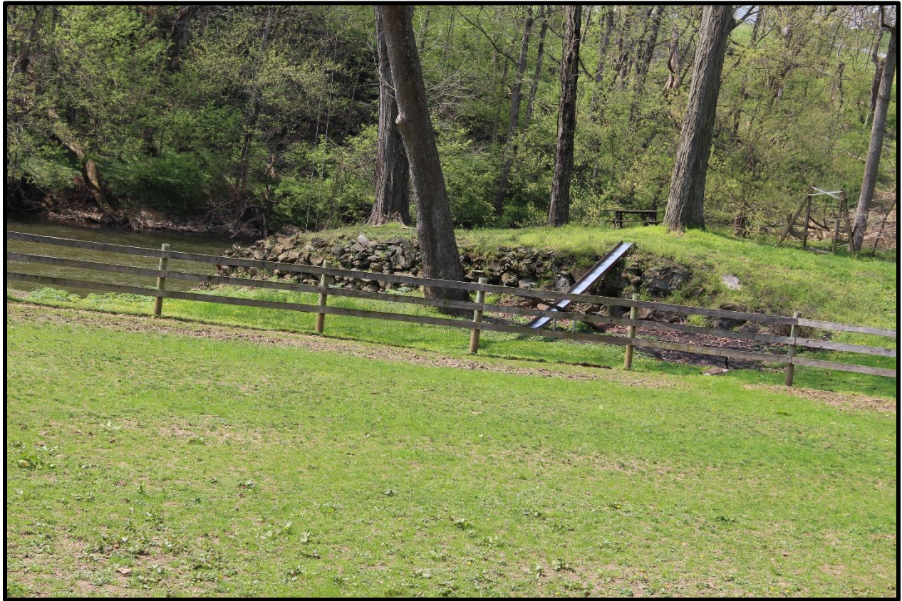
Photo 7: View of ruins of Lock No. 4 at Slackwater, Pennsylvania, facing east. View shows remnant of lock wall. Evidence from historic mapping indicates that Lock No. 4 was located south of Dam No. 4 at Slackwater, Pennsylvania and was accessed via a canal channel (Bare 1864:43).
