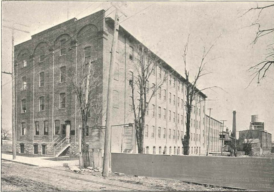
LANCASTER CORK WORKS (NEW ADDITION).
