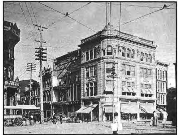
Watt and Shand Building
