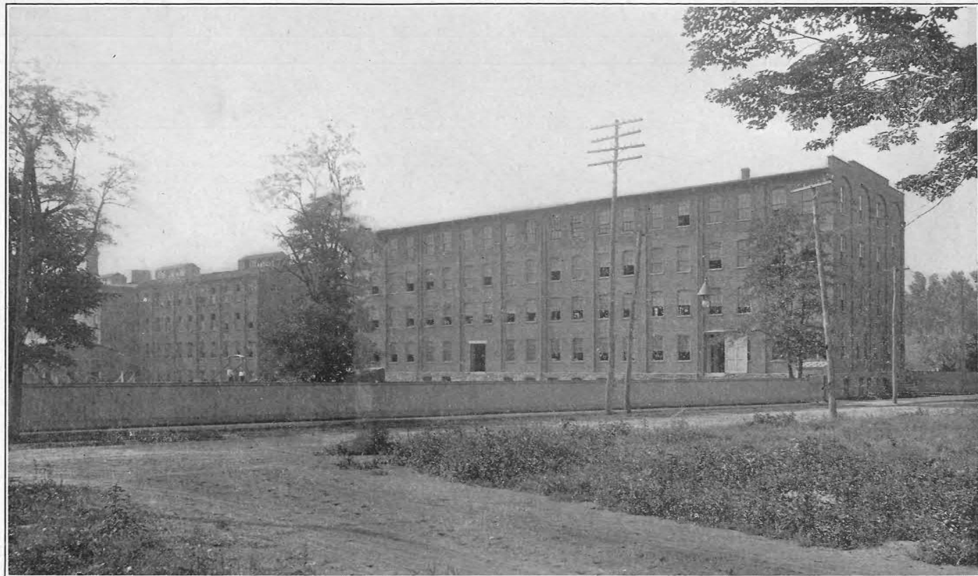
Armstrong Cork Works. 500 Employees. Opposite McGrann's Park Plot on New Holland Avenue.
