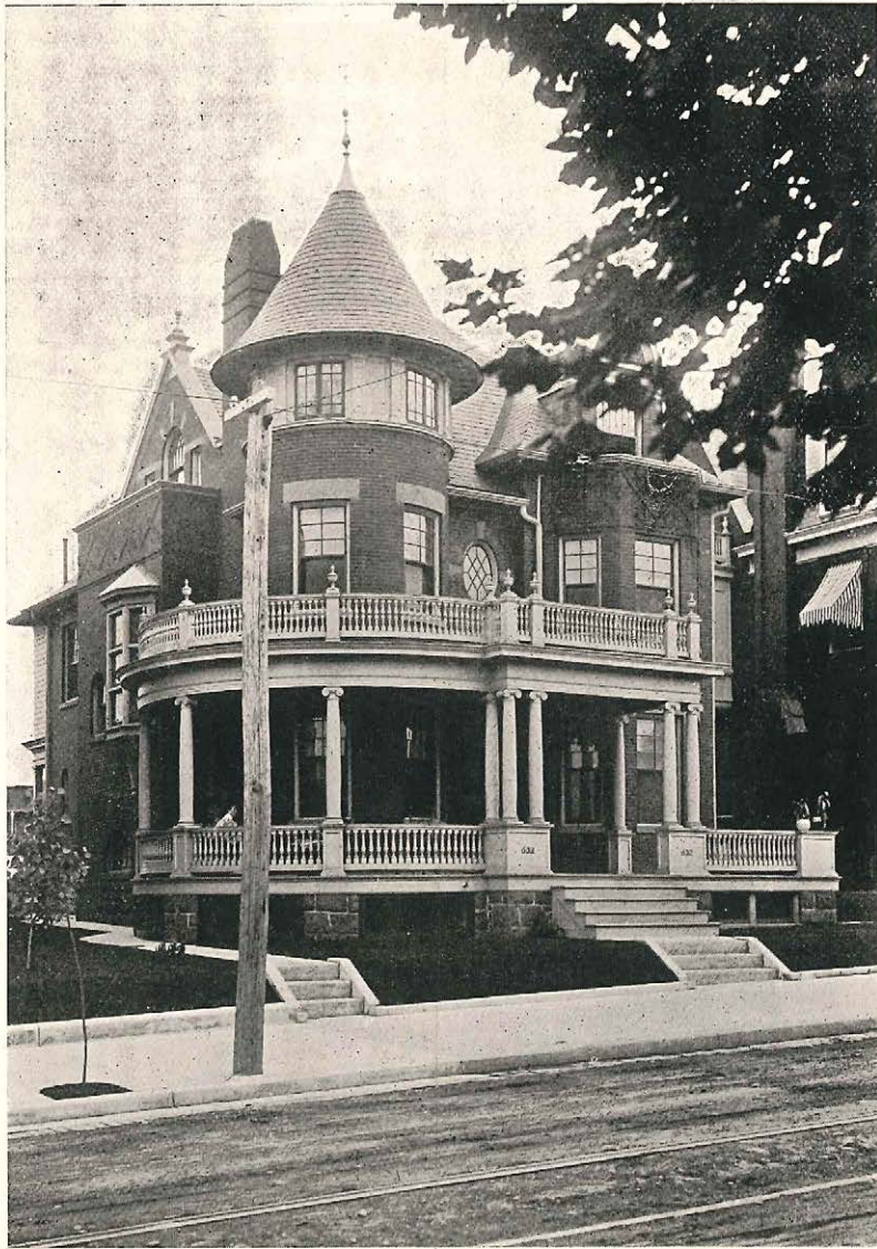
RESIDENCE OF MR. E. E. STEIGERWALT.
