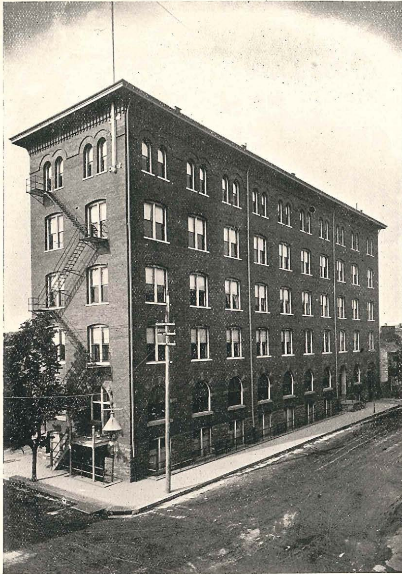
THE S. R. MOSS MANUFACTURING BUILDING.
