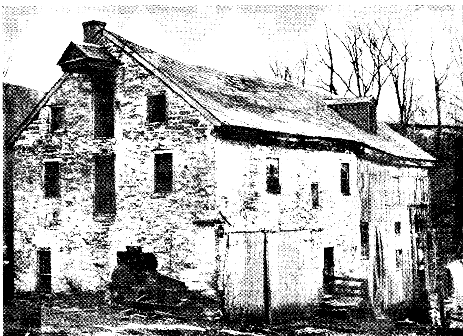
Eshelman's Mill on Mill Creek at its juncture with the Old Factory Road. Used as a gun factory by William Henry during the Revolution. Photograph by M. Luther Heisey, 1942.
