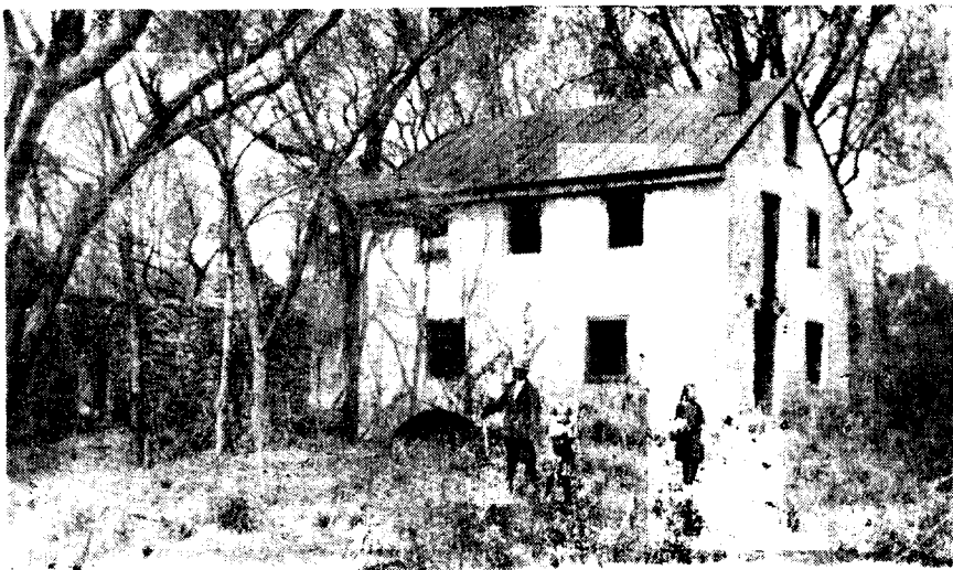
Henry Leman's Boring Mill located along Conestoga Creek opposite Pine-town (near Catfish, or Oregon). Forging, welding, planing and boring of rifle barrels were done here from the mid-1830's until 1850 when operations were moved to Lancaster and were powered by steam.
