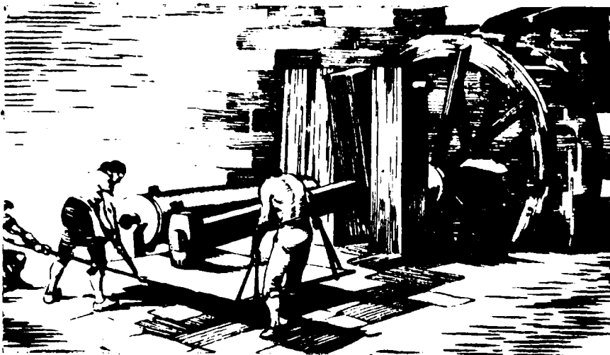
Water-powered tilt hammers worked charcoal iron plate in the numerous forges along the creeks of Lancaster County. The hammer from Speedwell Forge is exhibited in the Society's museum.
