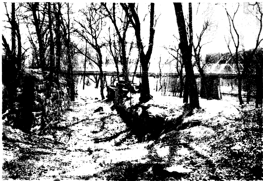
Lock No. 6 of Conestoga Navigation Company in 1958, one mile above mouth of creek; canal in operation 1828-1865.
