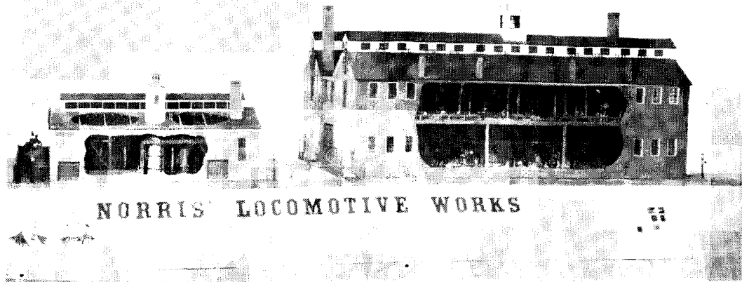
Model of Norris Locomotive Works, Philadelphia, on display in Smithsonian Institution. Structure at left is the foundry. Buildings at right include erecting shop, machine shop, finishing shop, and boiler shop.
