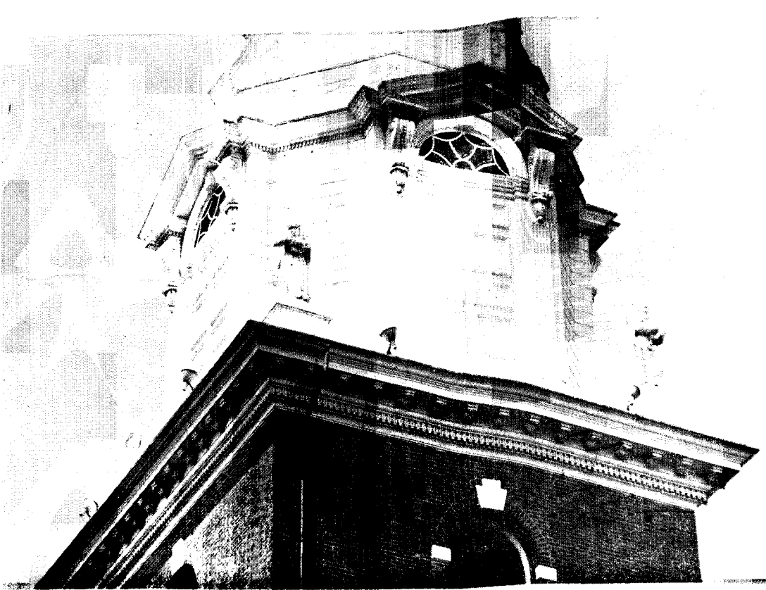
Detail of the lower steeple section of Trinity Lutheran Church.
