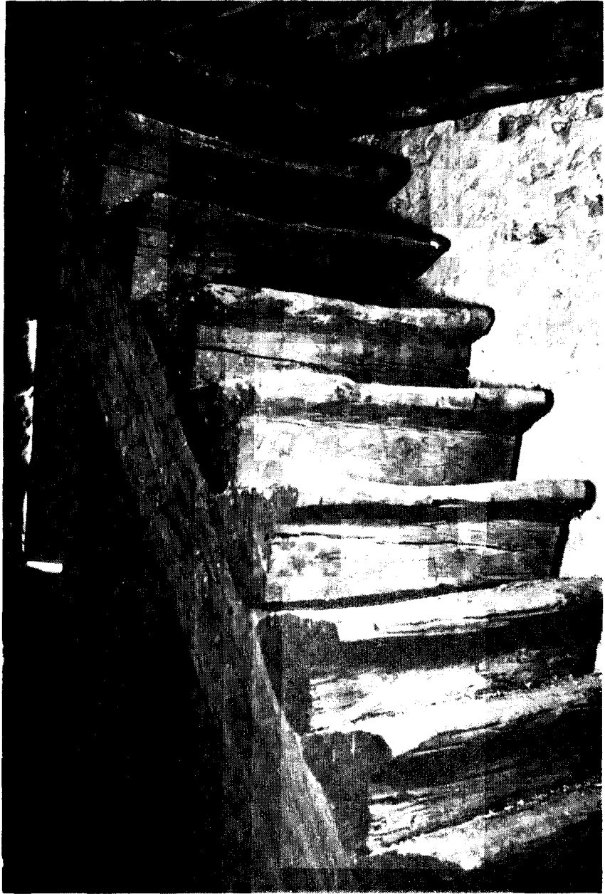
Original stairway between second floor and loft in Christian Herr house. Each step was hand-hewn from chunks of wood.
