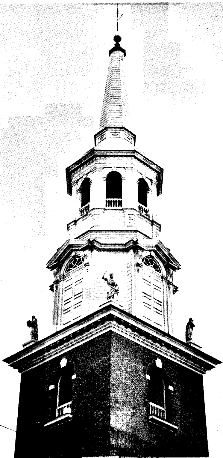
Detail of Trinity tower and steeple. Photo taken from the northwest.
