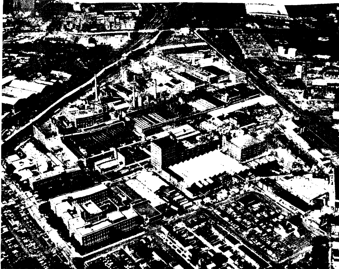
Lancaster Plant – Floor Division.
