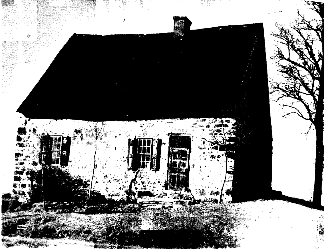
The Herr House before recent renovation.
