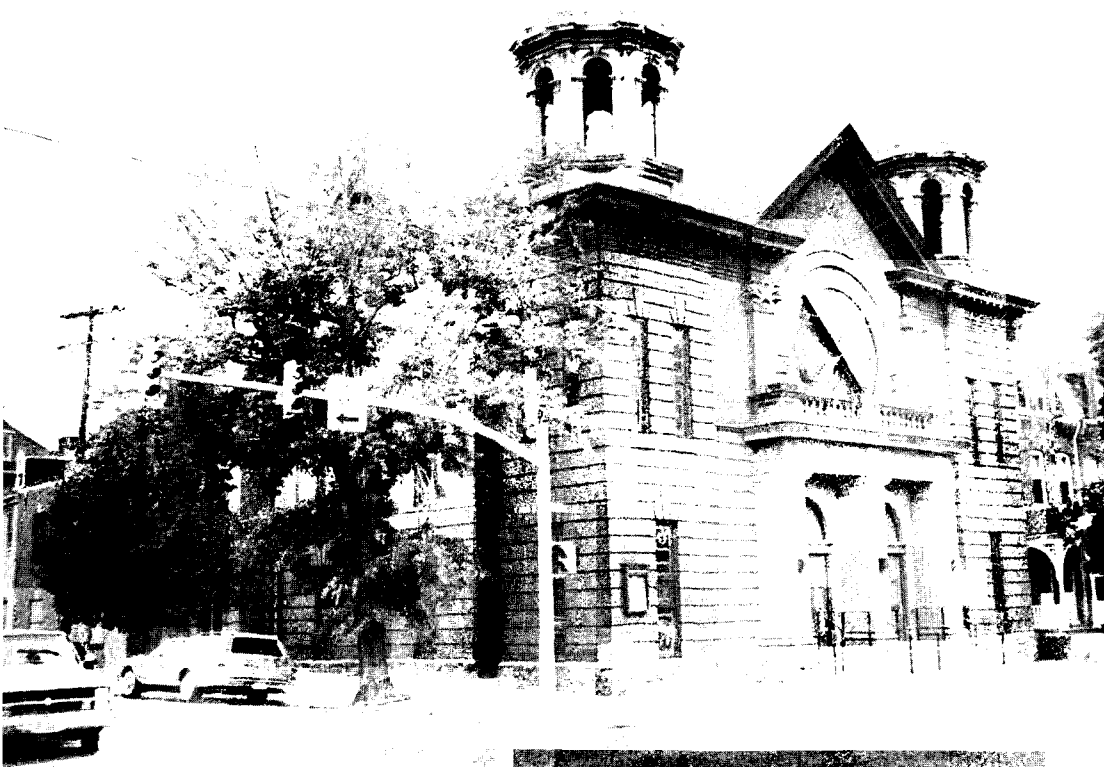
Temple Shaarai Shomayim at the northwestern corner of Duke and James streets is the house of worship owned by the Reformed Jewish congregation. It was built in 1895-6. The early synagogue was located at Orange and Christian streets 1867 to 1895. Congregation Shaarai Shomayim evolved from a German Jewish congregation chartered in 1856 to represent liberal or Reform Judaism. This house of worship is the fourth oldest still in constant use by American Jews.
