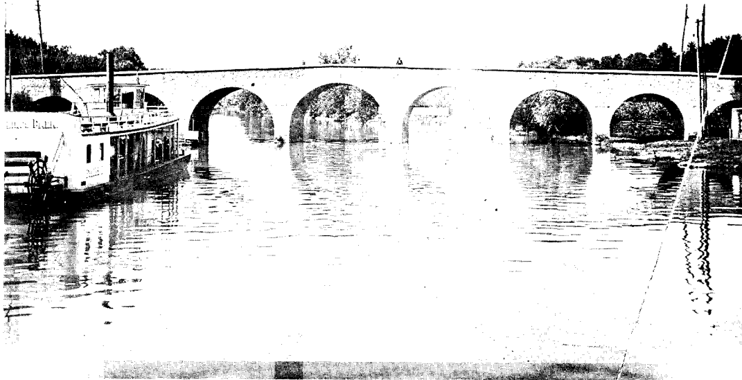
K. The nine-arch stone bridge known as Witmer's Bridge was built in 1800 by Abraham Witmer, replacing a wooden bridge he had constructed in 1788. It carried the Lancaster-Philadelphia traffic over the Conestoga River for 131 years until it was deemed too narrow for modern automobiles.
