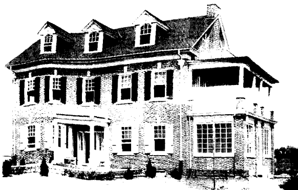
H. Roy Eshelman residence, northeast corner of North President and Buchanan Avenues, Lancaster.
