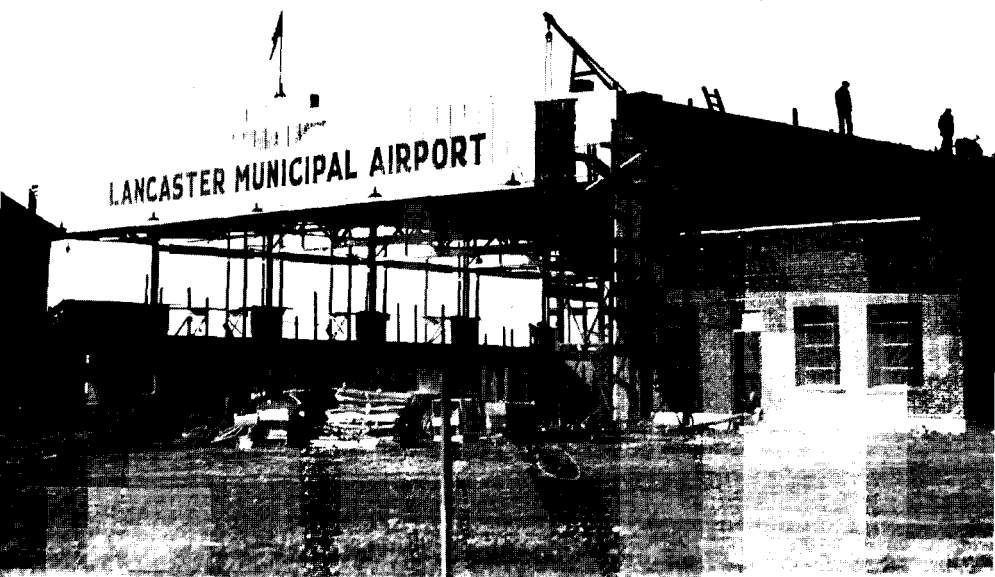
The main hangar of the new Lancaster Municipal Airport under construction in 1934. Construction was completed in nine months.
